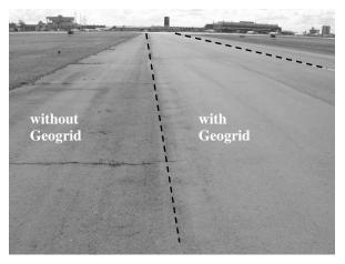
FIGURE 5 Overview of the Studied Section: View of the Taxiway to the Maintenance Hangar
