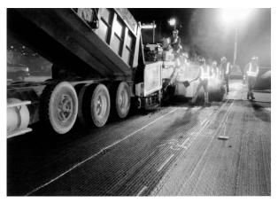
FIGURE 7 Installation of the Polyester Reinforcement Grid In 2000
