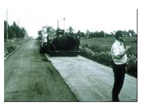
Figure 1. One of the first attempts to use a geogrid in asphalt pavement at the early 1970s
