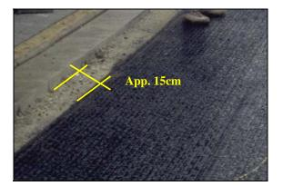
Figure 4. Fitted reinforcement (detail)
