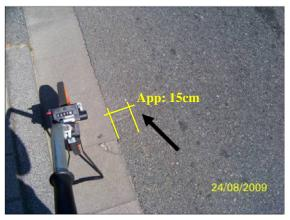
Figure 3. Lateral crack at the edge
