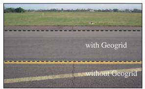
Figure 6. Joints of the concrete slabs reflect in the area where no reinforcement was used
