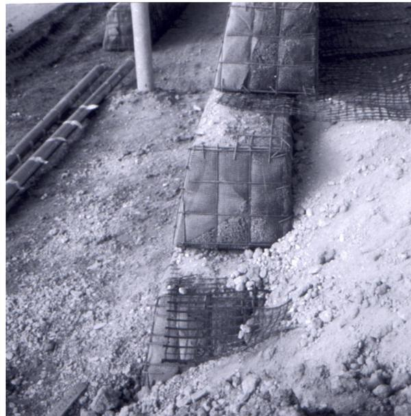
Figure 13. Unterkaka Logistics Centre: construction stage, PVA-geogrids, GeoGreen<sup>®</sup>-gabions, connections, fill soil
