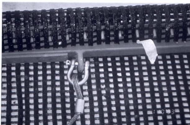
Figure 3. Tension bar used to tighten the aramid geogrid during installation
