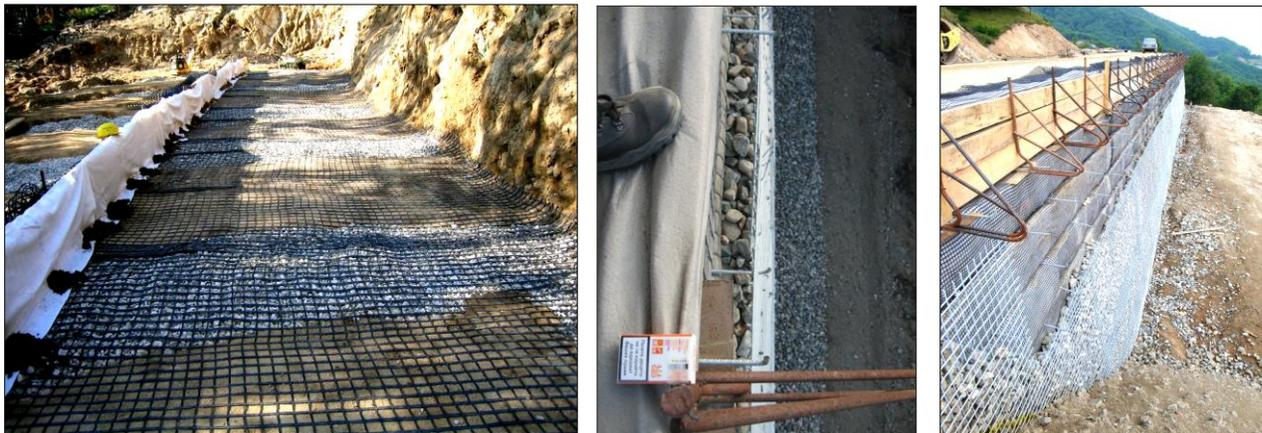
Figure 9. From left to right: wall base with drainage blankets, top view of stone-filled facing used, construction stages (formwork, geogrids, facing).
