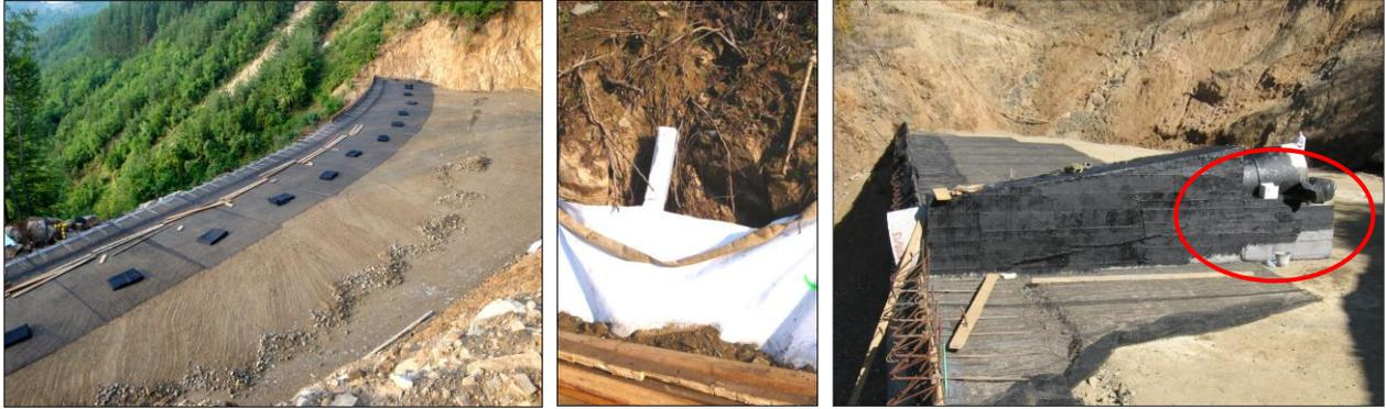
Figure 10. Pre-cut folded flexible geogrids waiting for installation, geotextile wick drain from rolled non-woven at the back of wall, culvert on geogrid-soil cushion.
