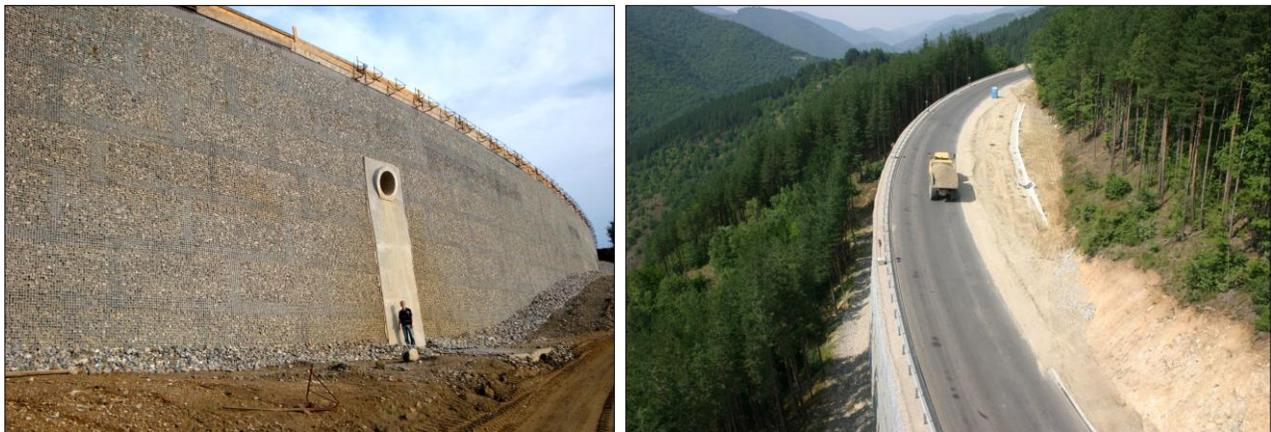
Figure 11. Front view of a GRS-wall before reaching the final height but with partially installed Muralex<sup>R</sup> facing and completed culvert (left), top view of a completed wall (right).
