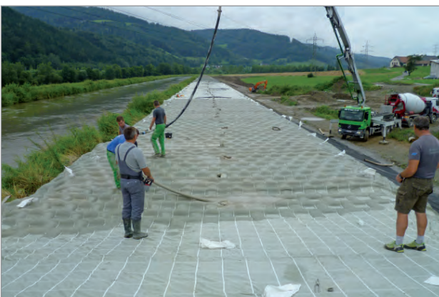
Filling Incomat ® with concrete
