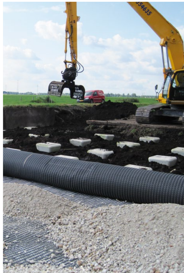
Geotextile reinforcement installed on piles (N 210; Netherlands)
